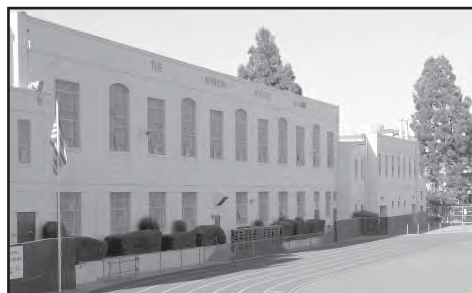
Konheim Athletic Building, scheduled to be demolished
