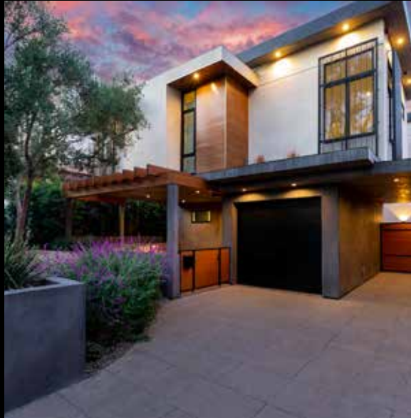
WEST HOLLYWOOD 9019 Elevado Avenue
