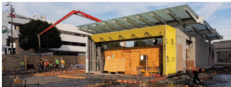
D LINE SUBWAY EXTENSION PROJECT Section 1 – Beverly Hills
