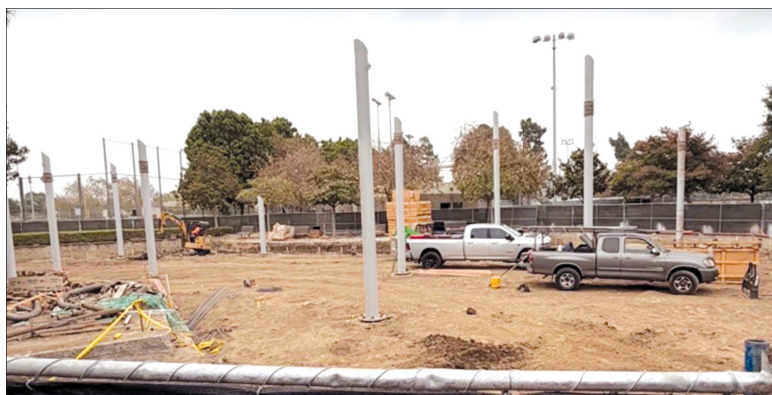
Construction Photo from June Staff Presentation
